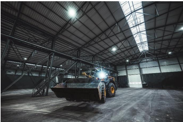
(2) Protected from the weather, around 8,000 t of material can be stored and treated in the 3,000 m 2 hall.
