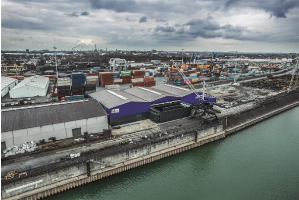
(1) The sliding roof on the port basin side enables direct transshipment from the hall to a ship or train.
